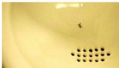
The fly turns into the black outline of a fly, etched into the porcelain. It improves the aim. If a man sees a fly, he aims at it. Fly-in-urinal research found that etchings reduce spillage by 80%.
